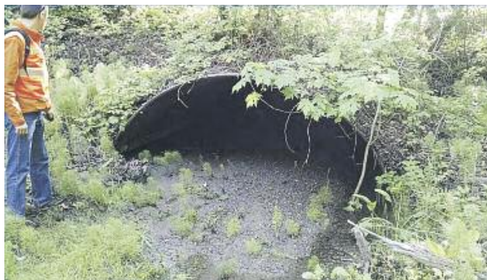
Las Trampas Creek crossing at Bollinger Canyon Road
